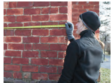
Historic Preservation student learning to record a historic building with measured drawings
